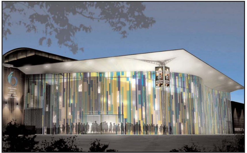
Construction of the newly-named Shenkmen Arts Centre will begin this fall next to the Orléans Client Service Centre. If all goes well it should be completed by the spring of 2009. File photo
