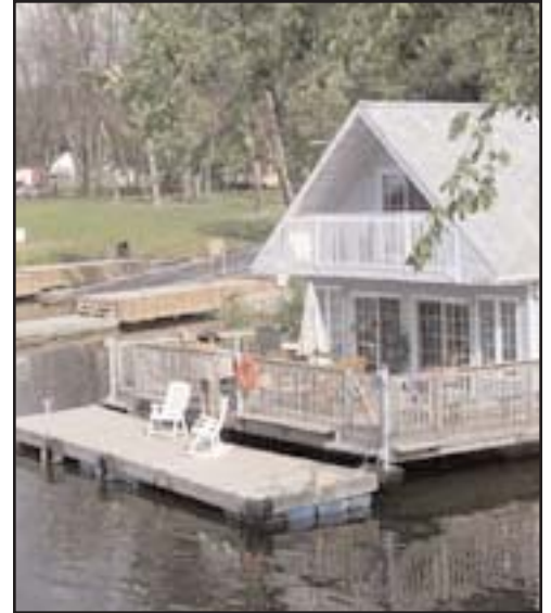
The Oziles house boat sits in front of the new boat ramp at the Petrie Island marina and tackle shop. File photo
